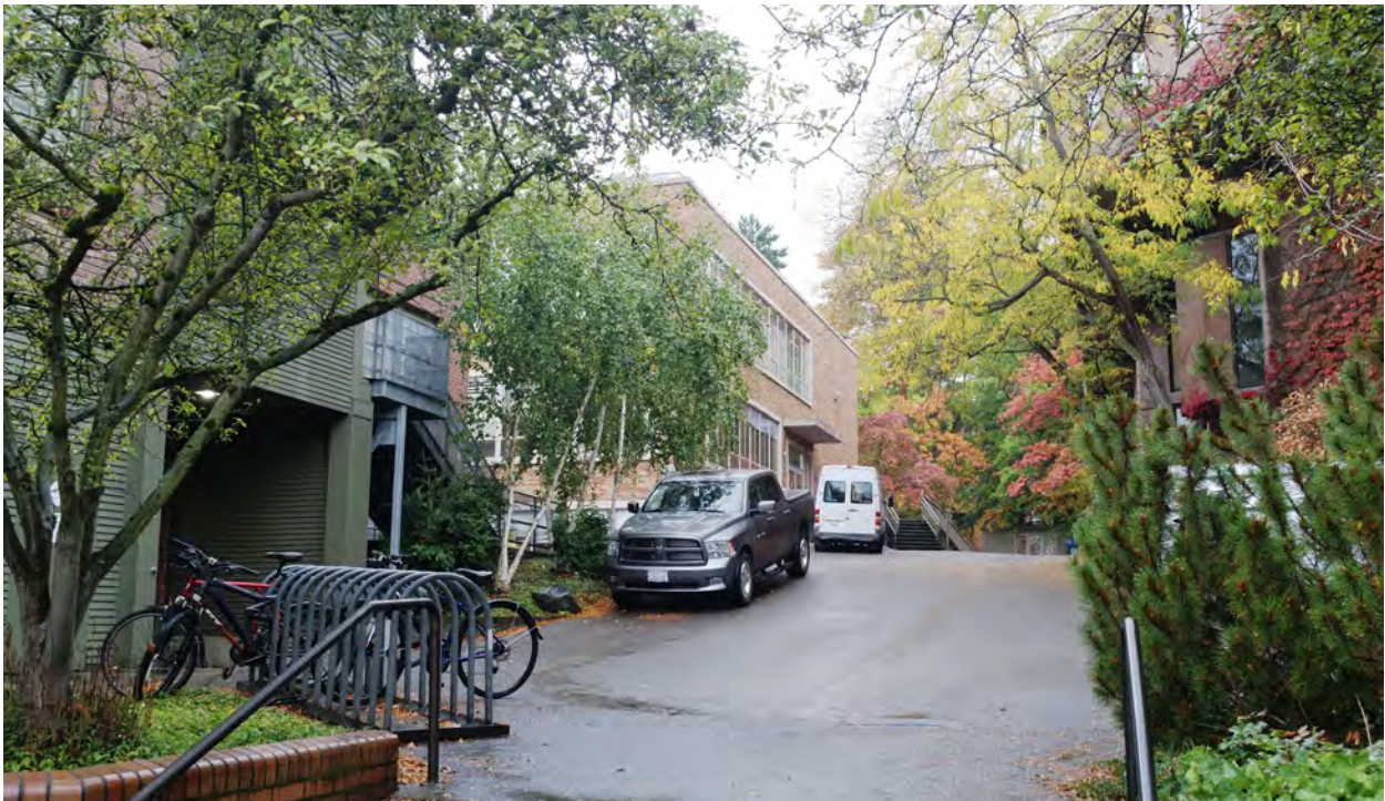
Figure 41. North passageway between the Engineering Annex (left), MEB (left, background), and Loew Hall (right), looking west.
