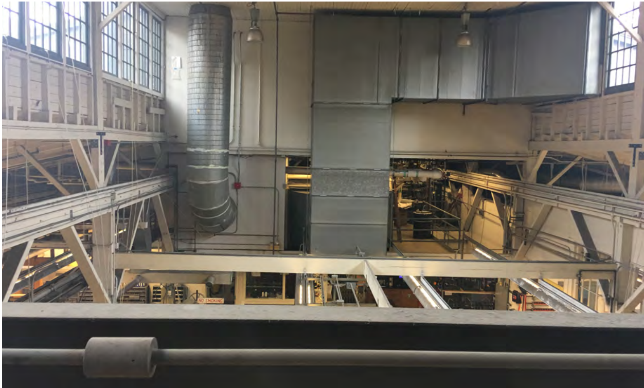
Figure 50. Main volume looking north from the mezzanine. The solid wall in the background is the original location of the wall separating the second floor from this area.
