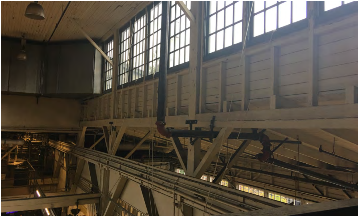
Figure 52. Main volume, looking northeast along the east facade.
