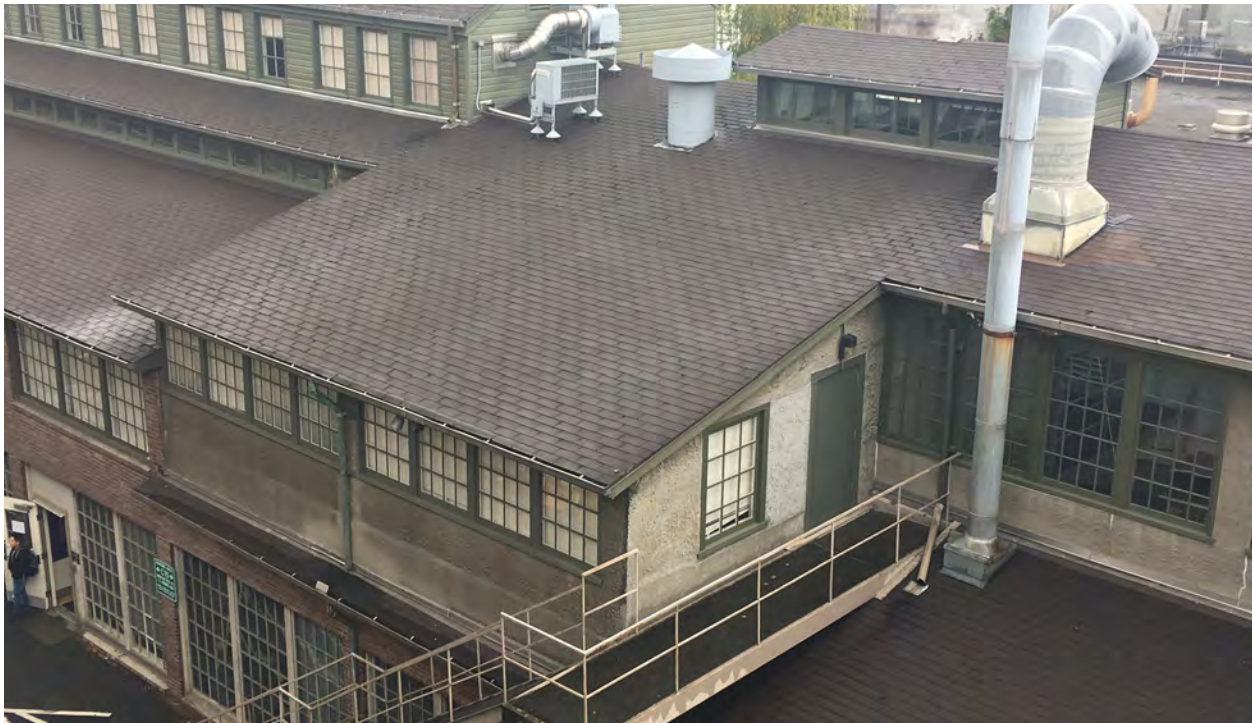
Figure 37. Looking northeast from the second floor of the MEB.
