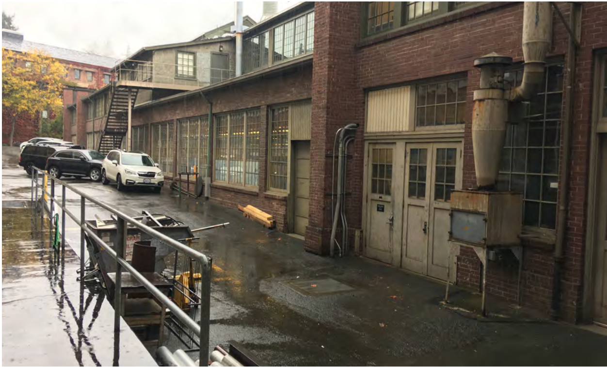
Figure 34. West facade looking north.
