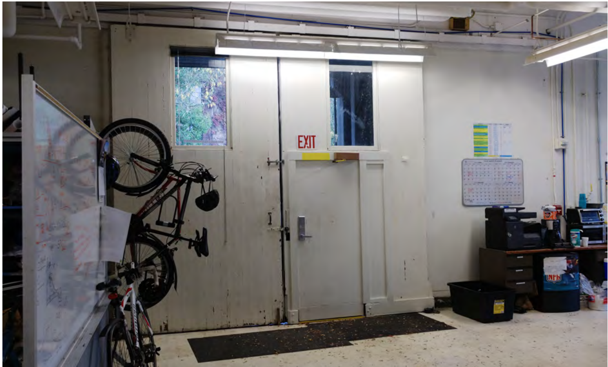
Figure 60. 1909 doors at the north end wall.
