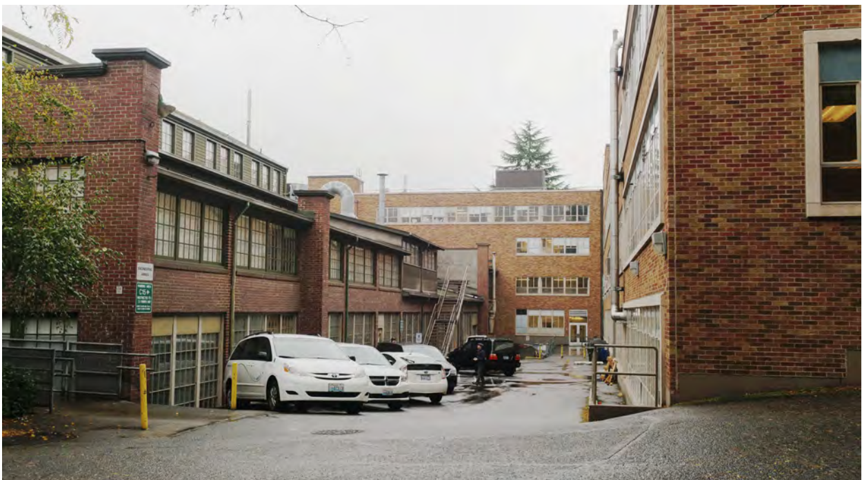
Figure 33. West facade looking south along the service court space. The Mechanical Engineering Building (MEB) is visible at right and across the south end of the service court space.
