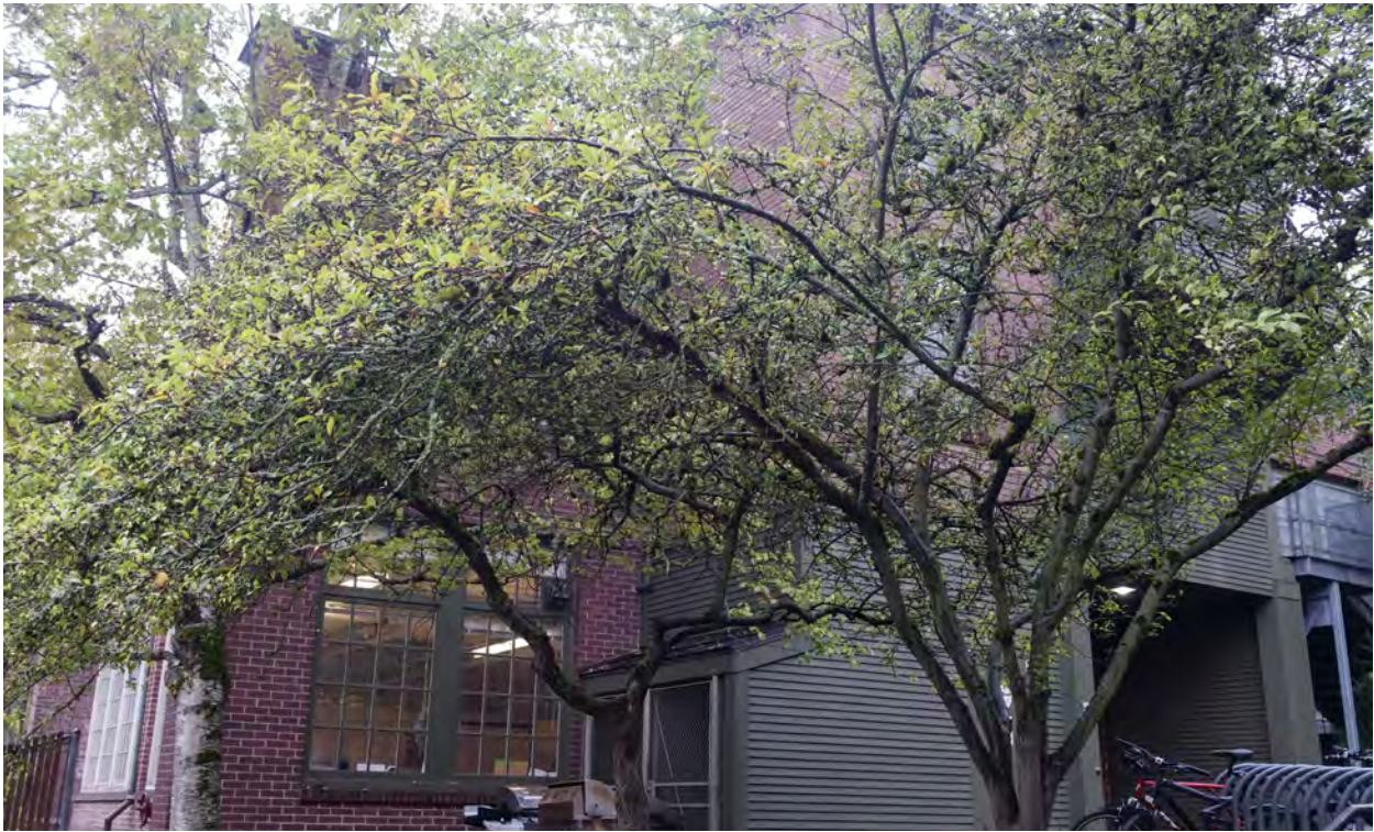
Figure 42. Northeast corner of the north facade.
