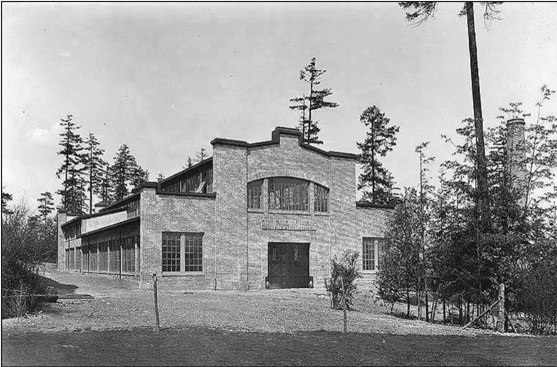
Above, exterior view of the Foundry Building in 1909. This view is looking north and shows the original south facade. The north and south facades were replaced in 1920 when the building was expanded, with a similar appearing end walls. The original north facade was encapsulated later by a two-story extension of the building. The extension abutted and was internally linked at the second floor with the new Mechanical Engineering Building in 1959.
