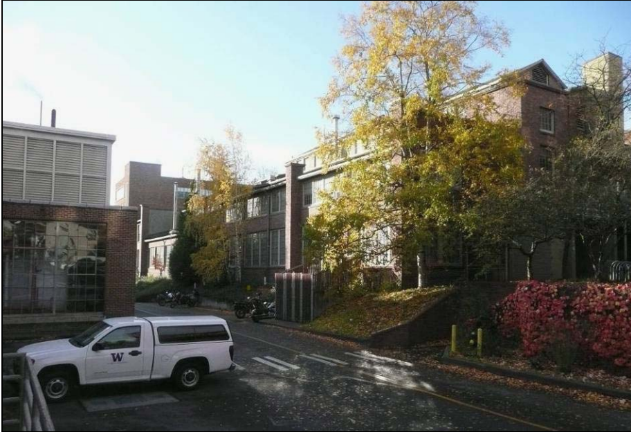
Above: Context view of looking south on Jefferson Road with the Power Plant to left (east).
