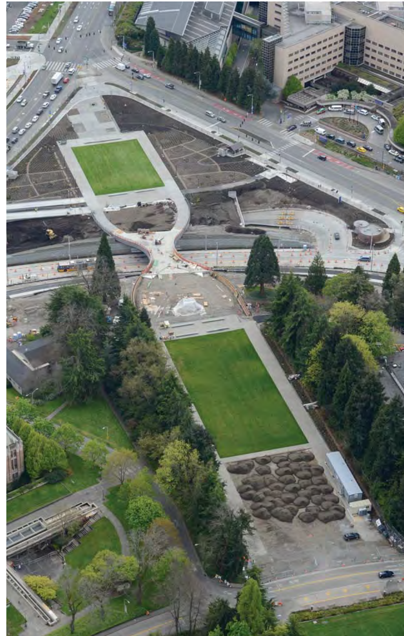
RAINIER VISTA CONSTRUCTION 2015
