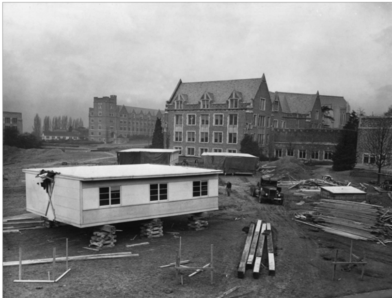
CONSTRUCTING BARRACKS NEXT TO FROSH POND
