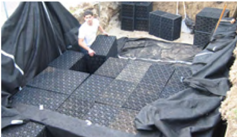
SUBSURFACE GEOGRID INSTALLATION
