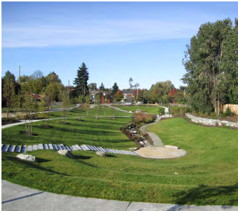
MADISON VALLEY STORMWATER OVERFLOW FACILITY
