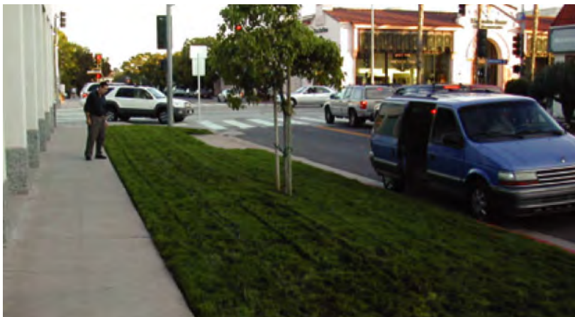
FINAL APPEARANCE OF GEOGRID INSTALLATION
