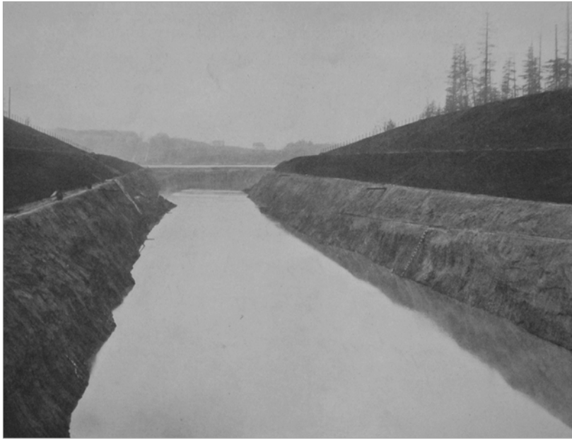
MONTLAKE CANAL UNDER CONSTRUCTION, 1915
