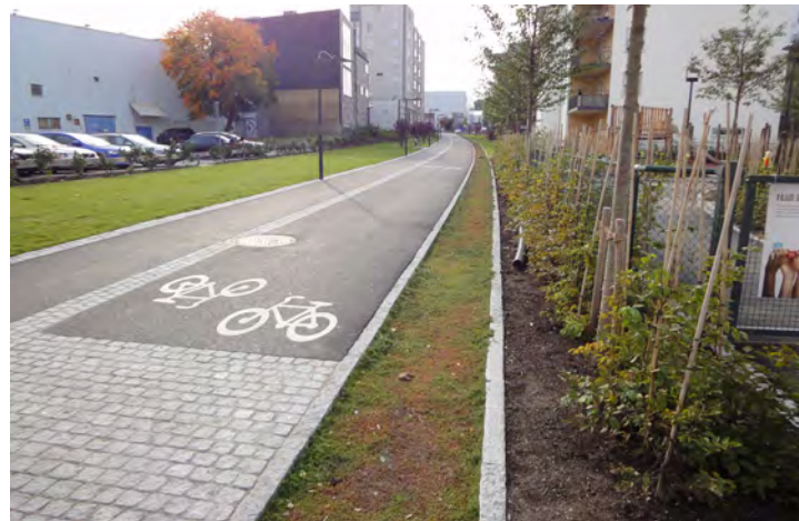
SAND FILTER ALONG A BIKE PATH IN COPENHAGEN
