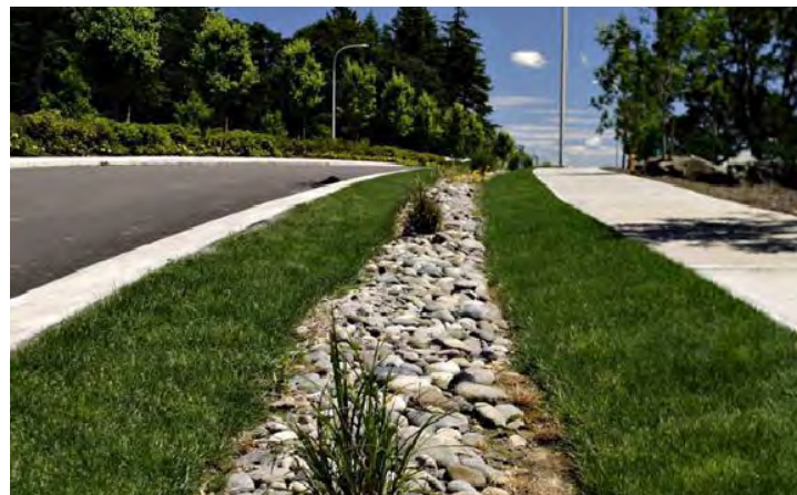
GRAVEL FILTER IN EAGLE LANDING. OR
