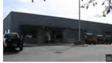
Physical Plant Building
