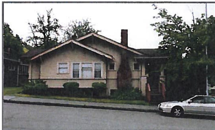
Field site no. 3 side (north) facade view. Source: Artifacts Consulting, Inc. 2008.
