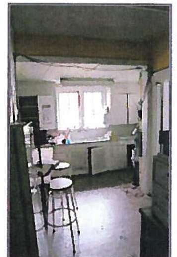
Field site no. 2 kitchen space looking west. Source: Artifacts Consulting, Inc. 2008.
