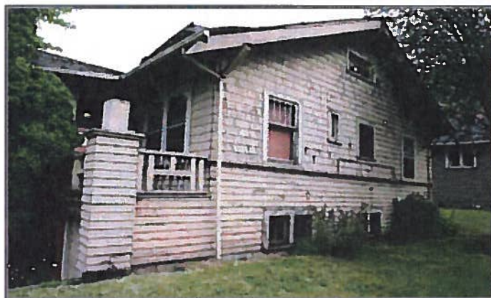
Field site no. 3 partial front (west) and side (south) facade view. Source: Artifacts Consulting, Inc. 2008.
