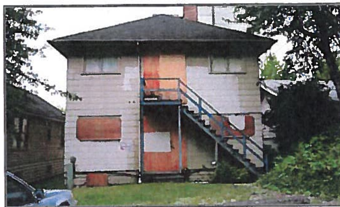
Field site no. 5 rear (east) facade view. Source: Artifacts Consulting, Inc. 2008.
