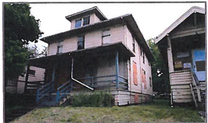
Field site no. 5 front (west) and side (south) facade view. Source: Artifacts Consulting, Inc. 2008.
