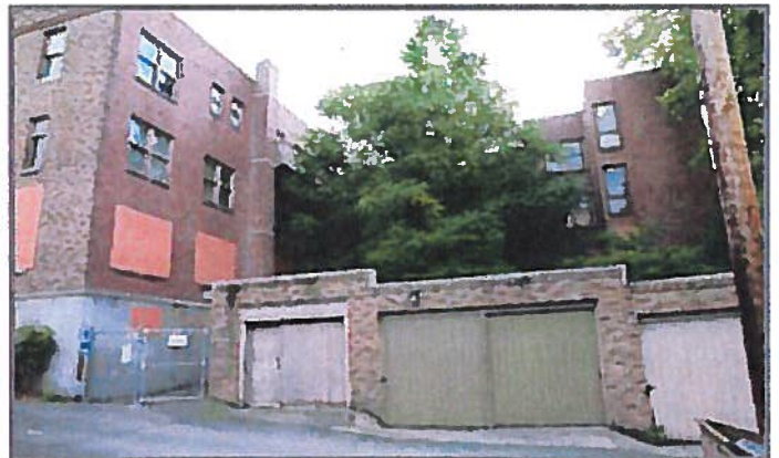
Field site no. 1 rear (west) facade view. Source: Artifacts Consulting, Inc. 2008.
