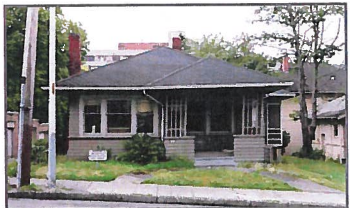
Field site no. 2 front (north) facade view. Source: Artifacts Consulting, Inc. 2008.
