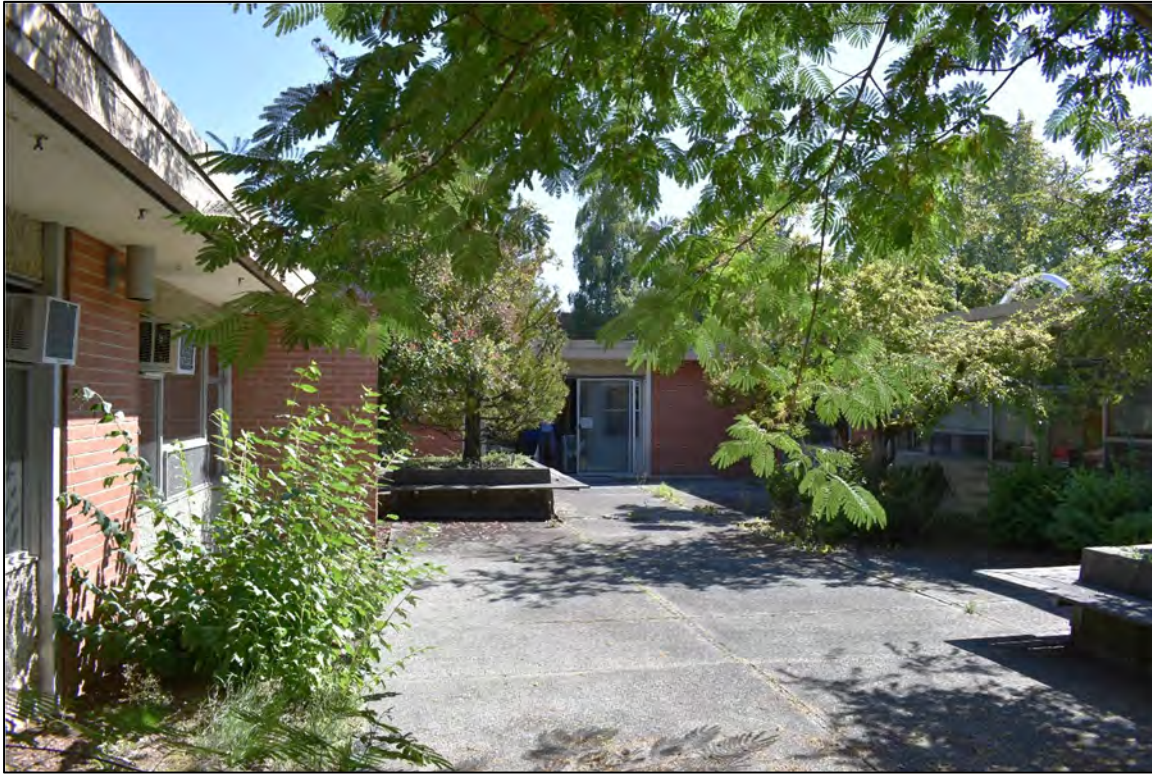
Small interior courtyard, view south.
