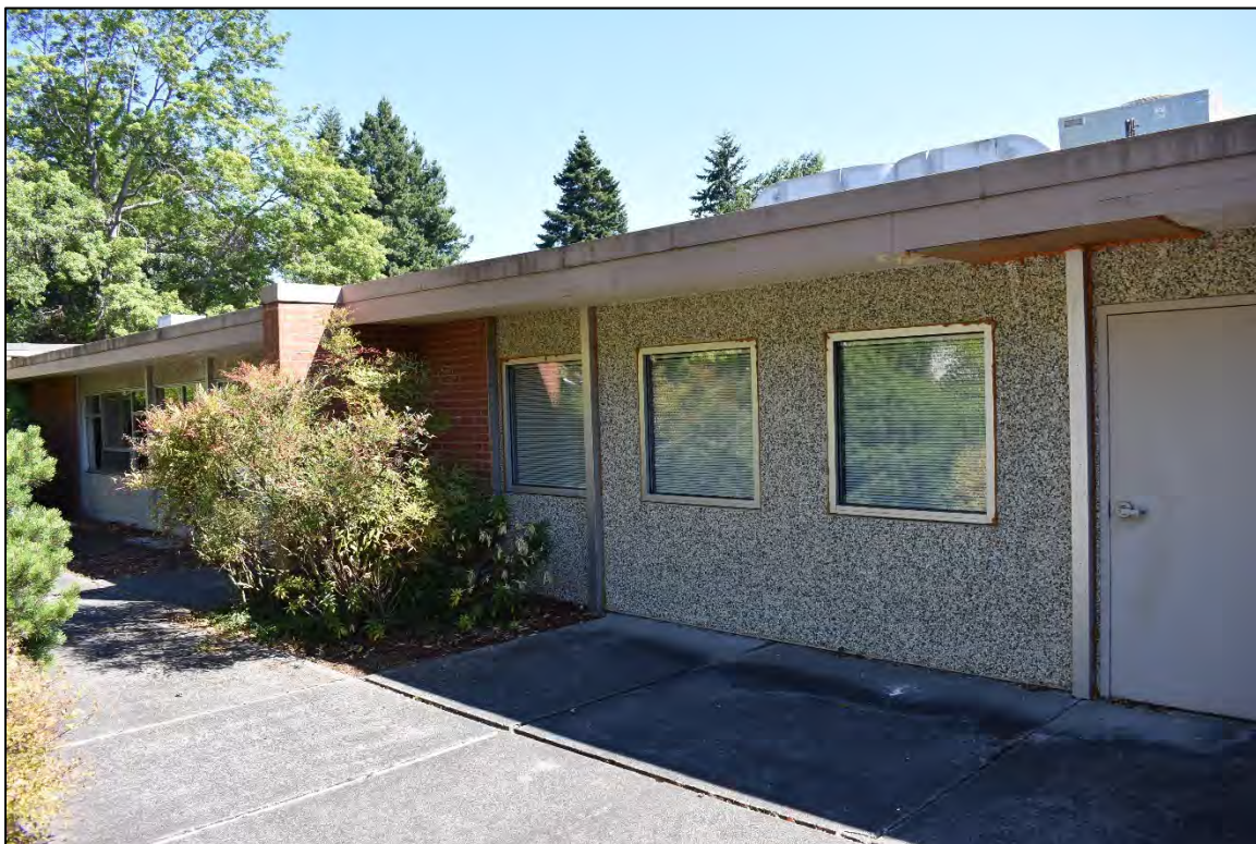
North elevation on exterior courtyard.
