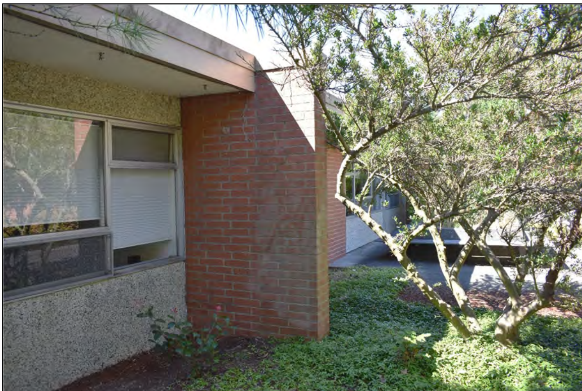
Large interior courtyard, detail of soffit, windows, and fin wall.
