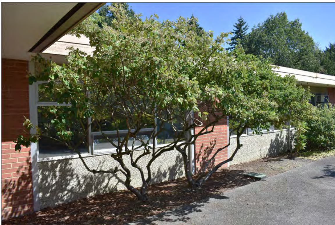
Large interior courtyard, view east.
