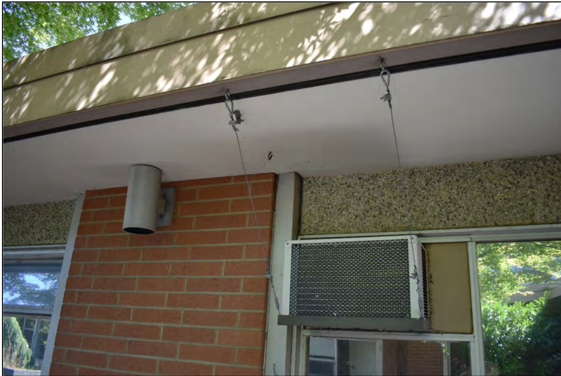
Large interior courtyard, detail of soffit and wall.
