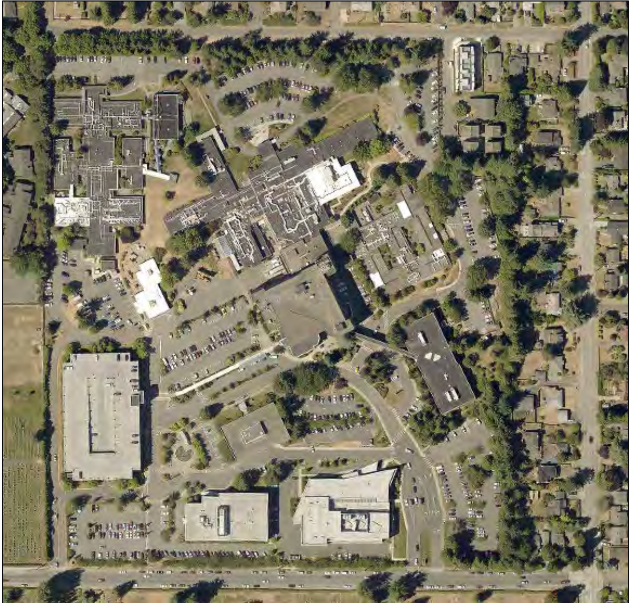
Aerial photo of the Northwest Hospital campus c.2018 without annotations; north is up. (KCTA)
