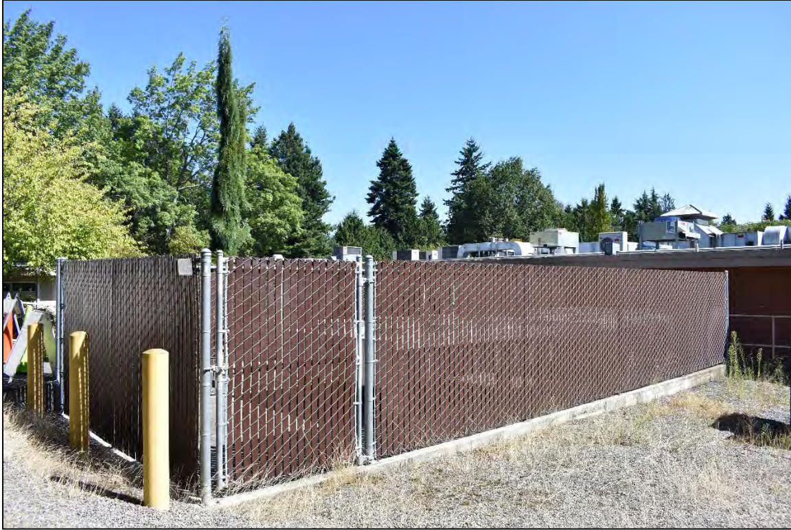
Equipment area on north elevation.
