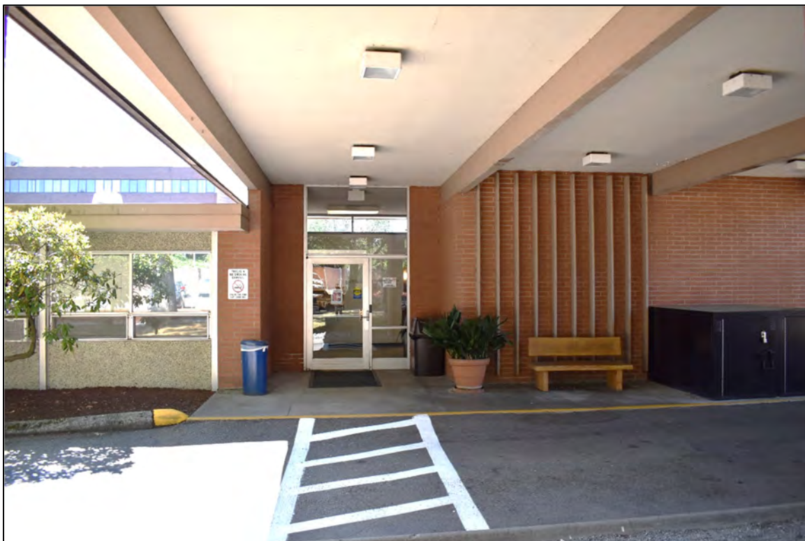
Front (east) entrance to building.
