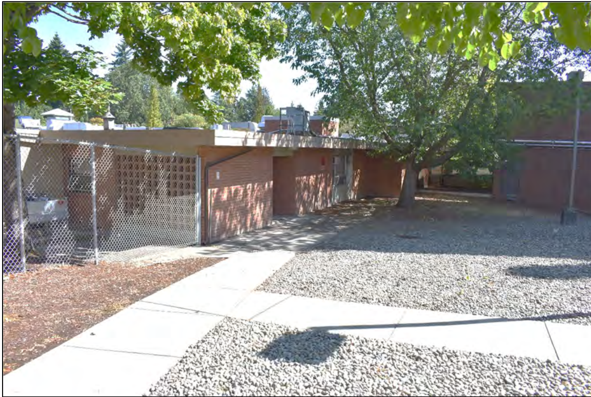
Partial west elevation, view south.
