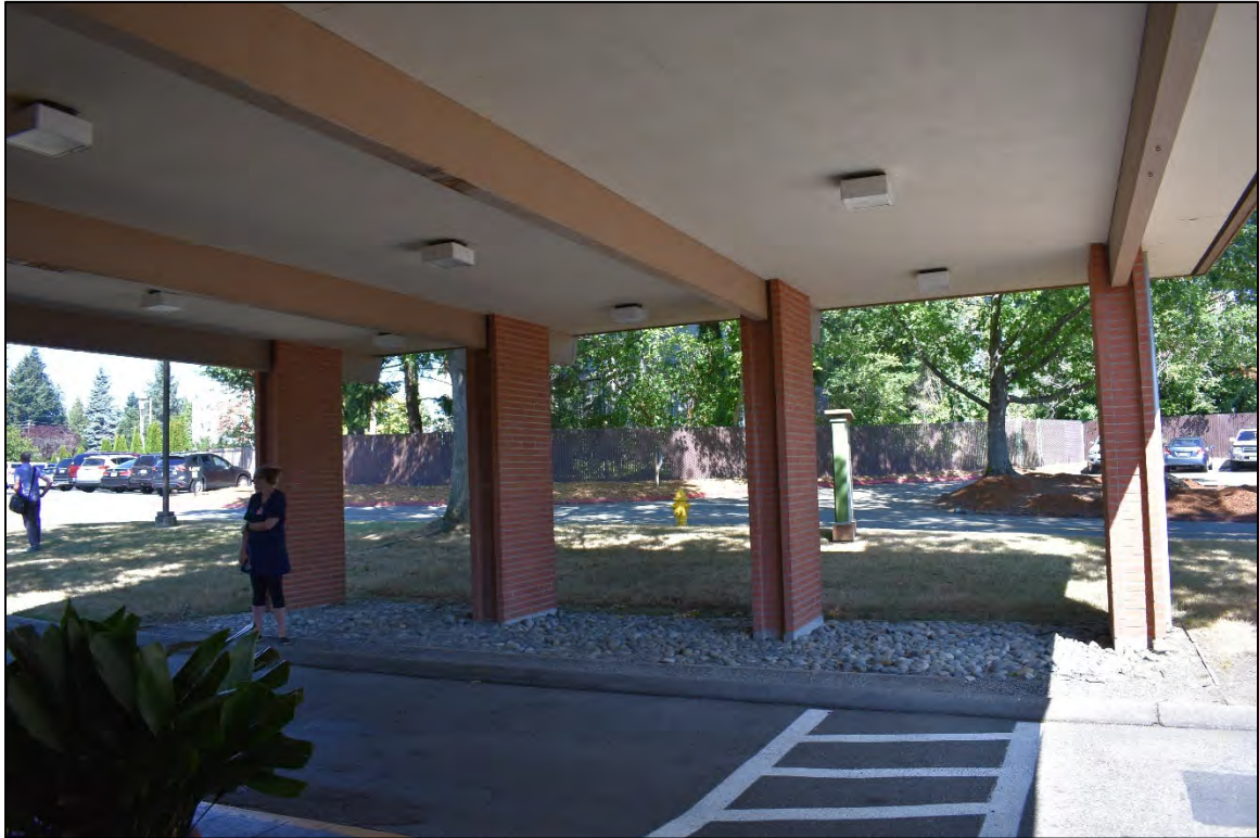
View east from front entrance to building.
