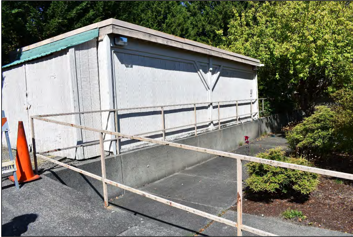
Shed/garage on north edge of exterior courtyard.
