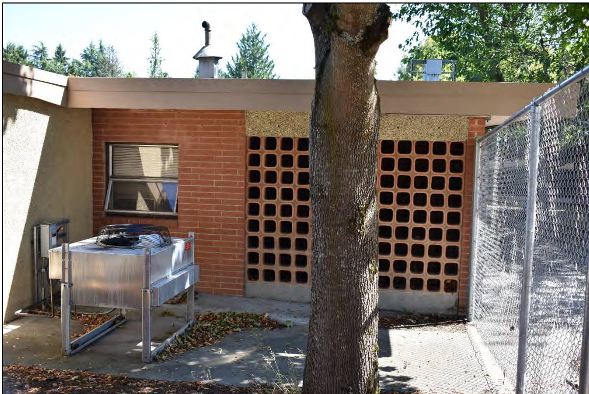
Area inside fencing on west elevation.
