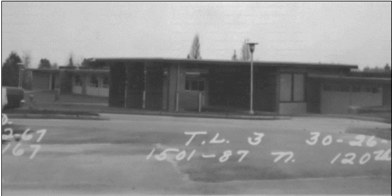
1967 view of the subject building, showing drop-off/porte-cochere on east elevation. Detail view of very poor original tax assessor photo. (KCTA)
