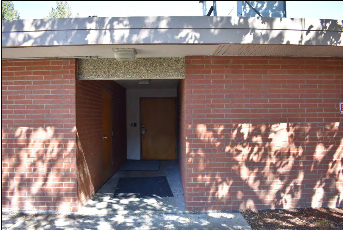
Service entrance on west elevation.
