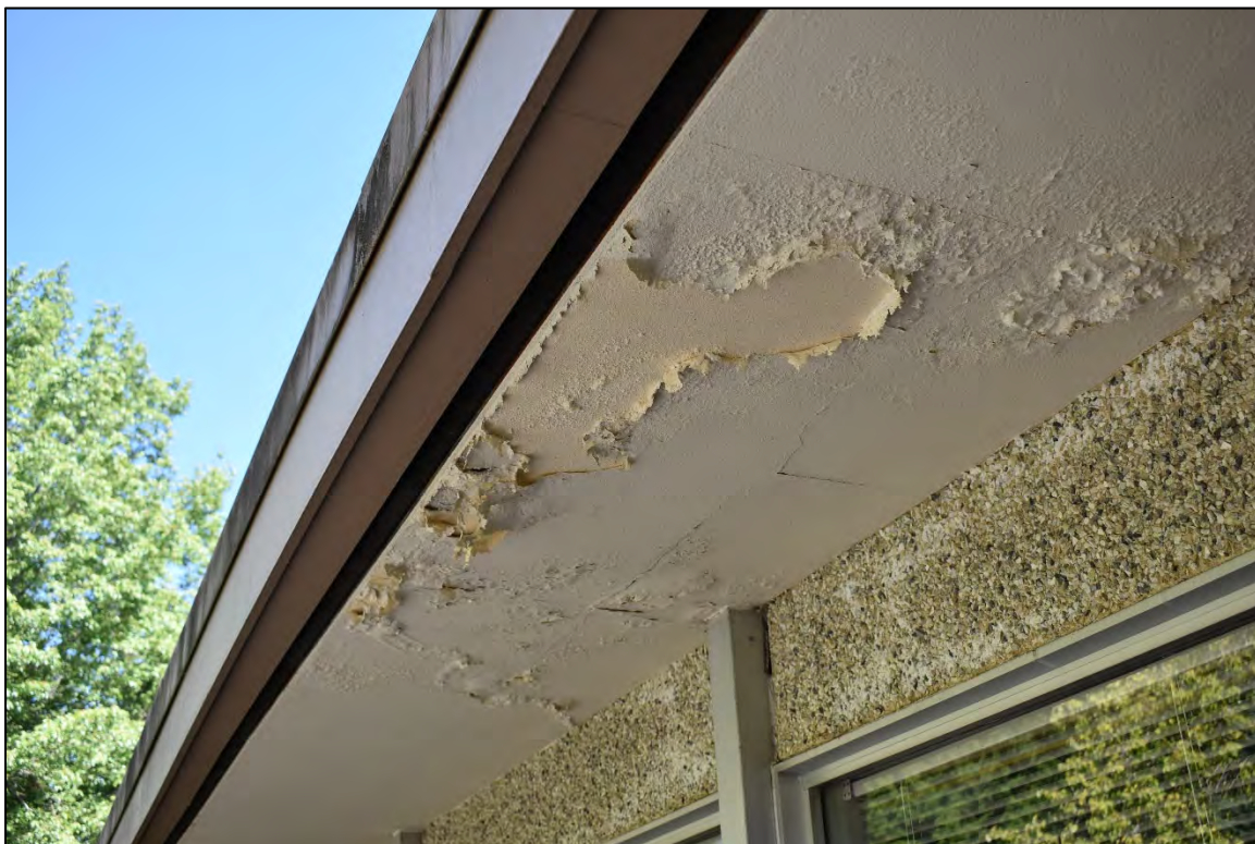
Exterior courtyard, detail of soffit.
