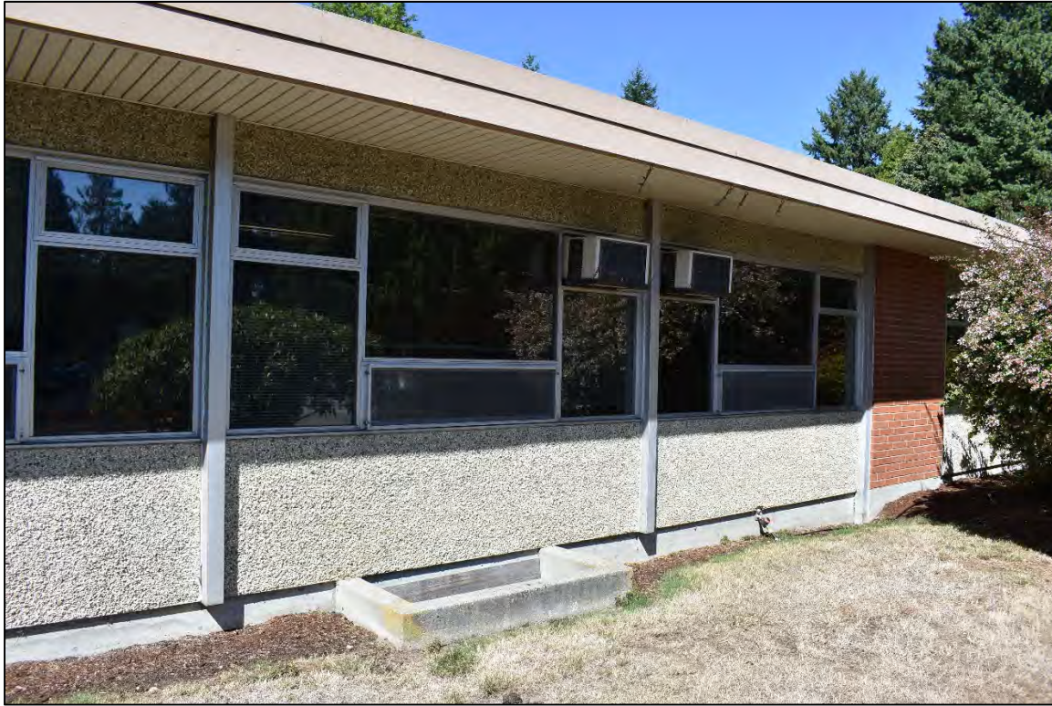
South elevation, view east.
