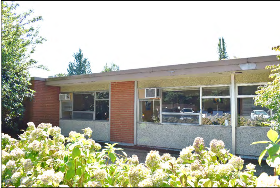
East elevation, view south.
