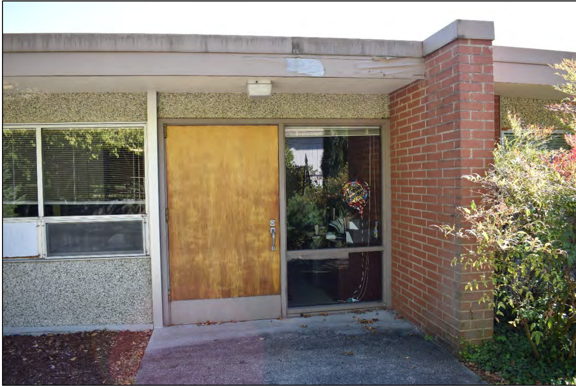
Exterior courtyard, detail of door on north elevation.
