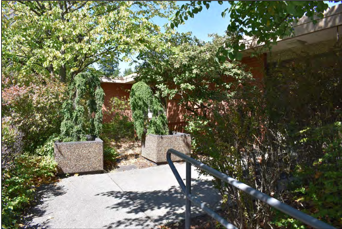
West elevation, west entrance.
