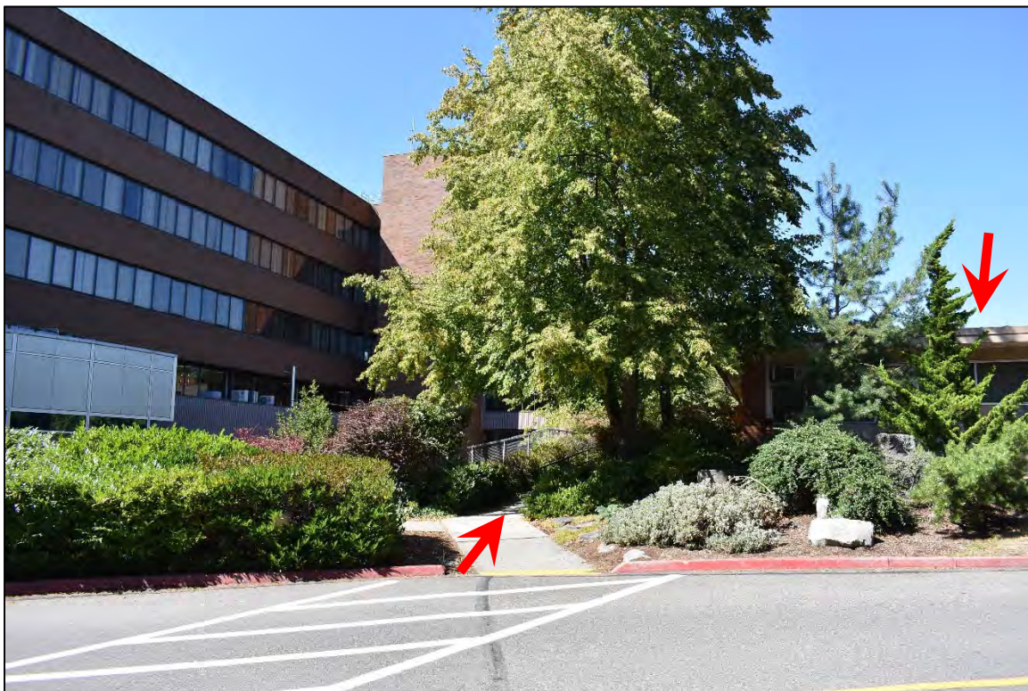
Context: West entrance, northwest view; subject building indicated by arrows.
