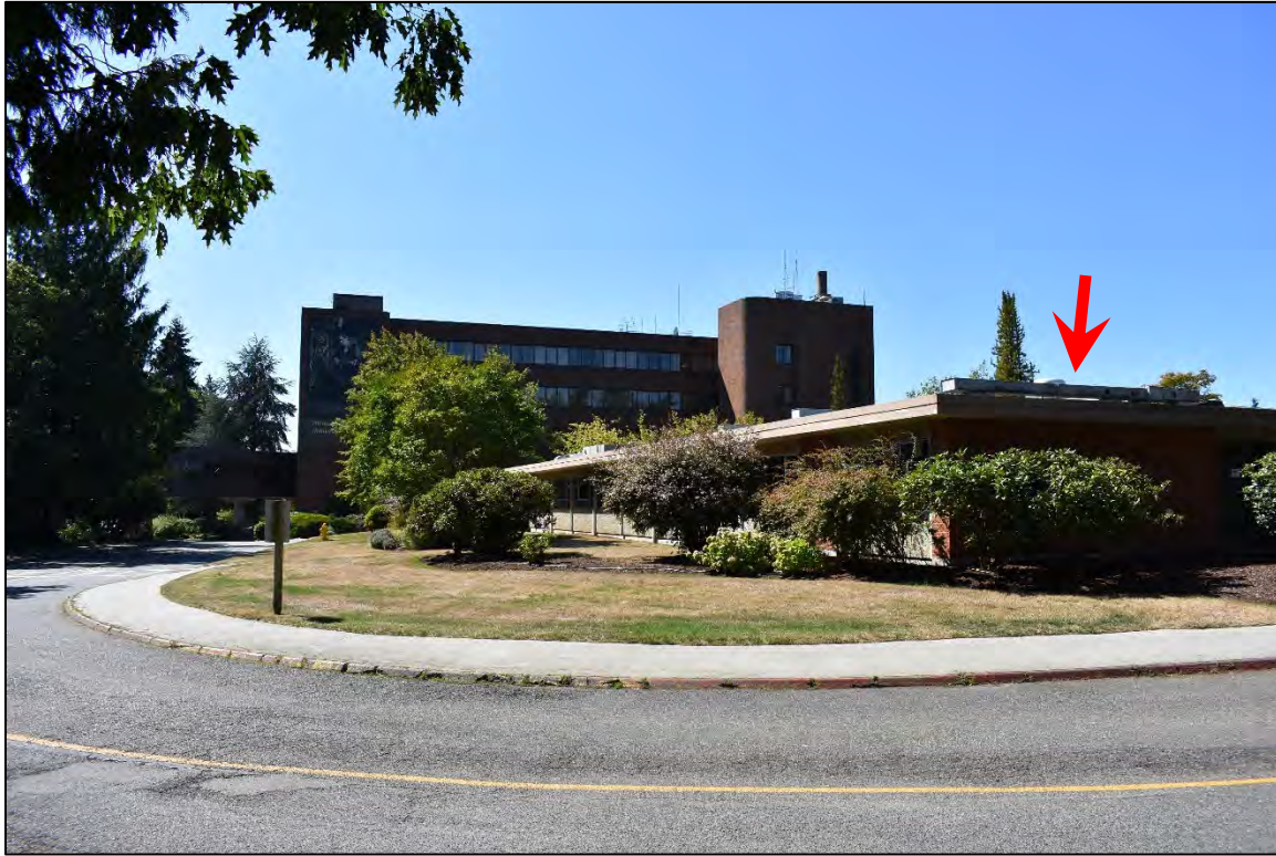
Context: view west, subject building indicated by red arrow.
