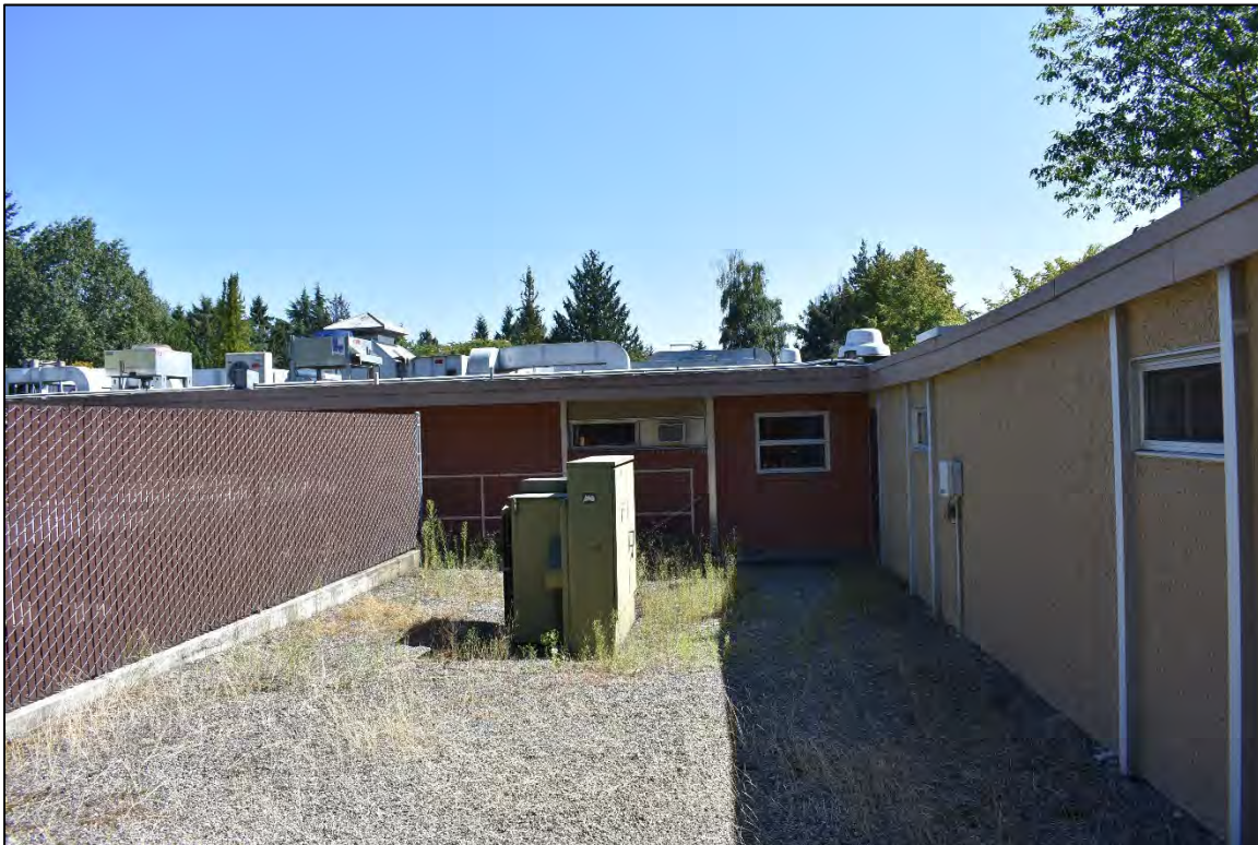
Equipment area on north elevation. Building element at right is the remaining stub of the original enclosed walkway (largely demolished c.2005) which connected the subject building to the B-Wing.
