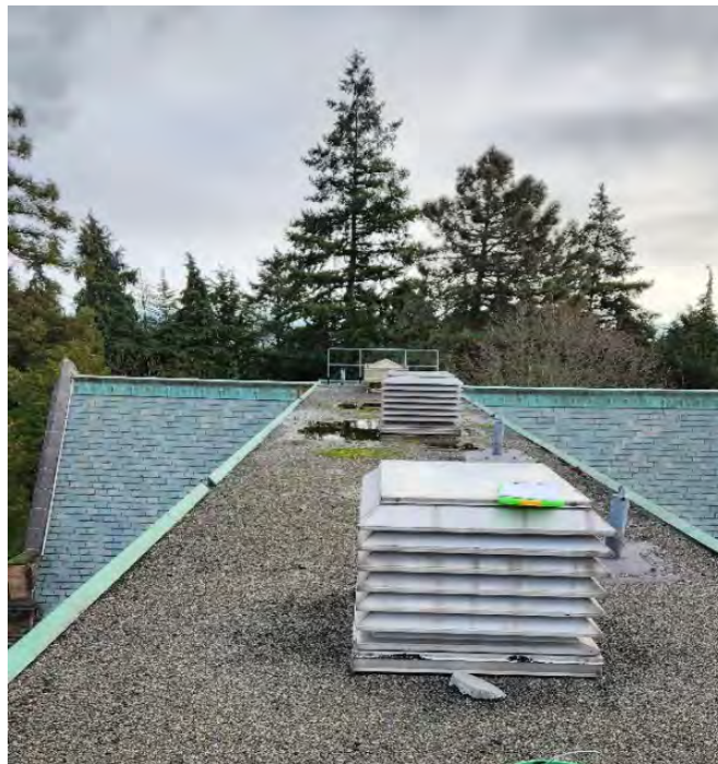
Photo 10: ACM containing silver and black exhaust sealant. ACM built up roofing.
