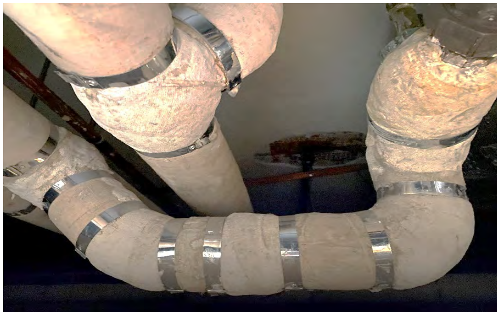
Photo 6: ACM hard fittings and elbows above dropped ceiling throughout building.
