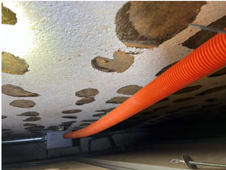
Photo 3: 12" tile with black ACM mastic underneath carpet. Beige and white/off-white 12" tile and black ACM mastic throughout the ground, first and second floor.
