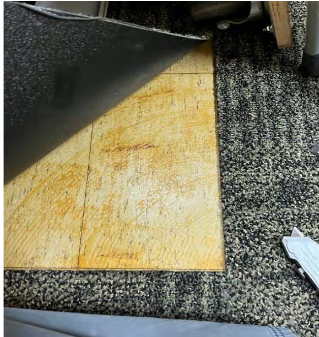
Photo 3: 12" tile with black ACM mastic underneath carpet. Beige and white/off-white 12" tile and black ACM mastic throughout the ground, first and second floor.
