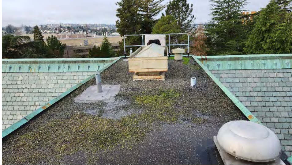
Photo 11: ACM black roof patch, ACM built up roofing.
