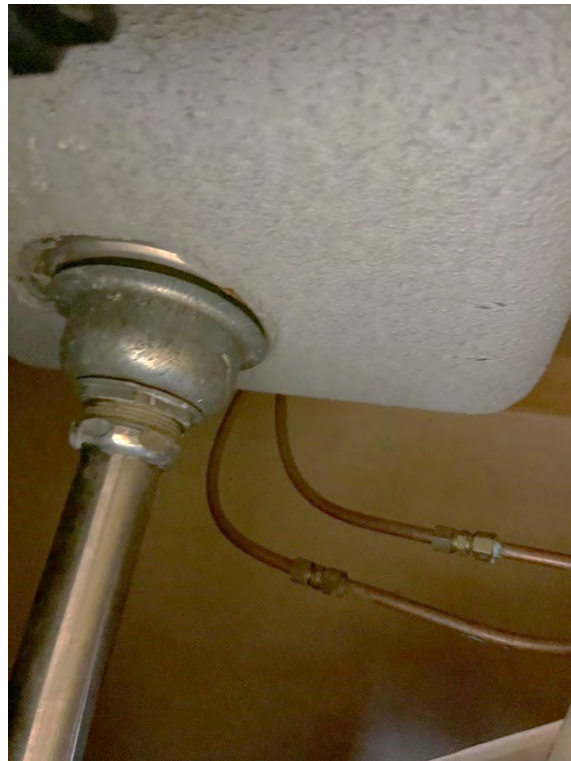
Photo 8: Off-white ACM sink undercoat room 107H.
