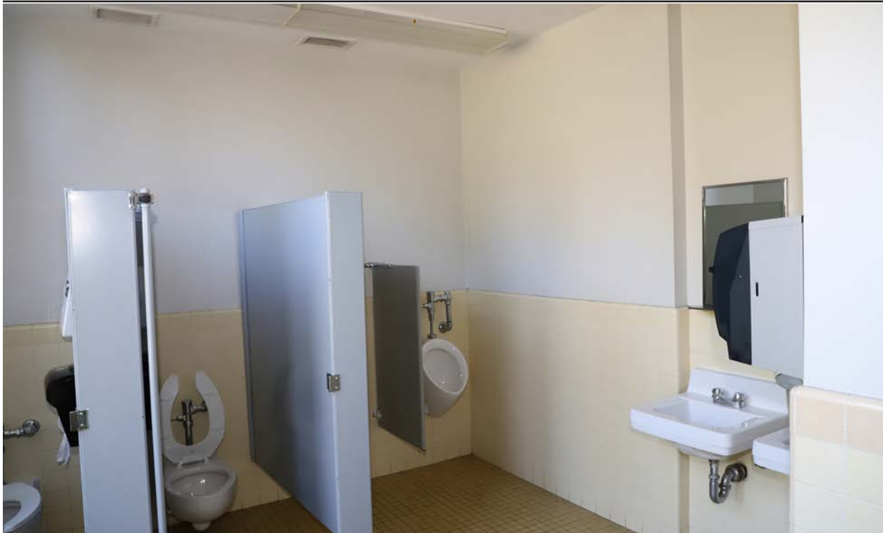
Figure 45. Second floor restroom, typical configuration.
