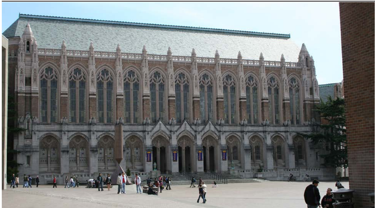
Figure 80. 2009 view of Suzzallo Library.
