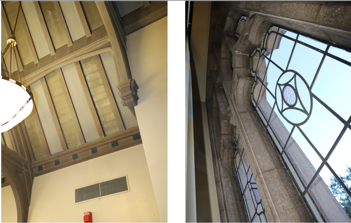
Figure 57. Lecture Hall, ceiling detail (left) and north window detail (right).
