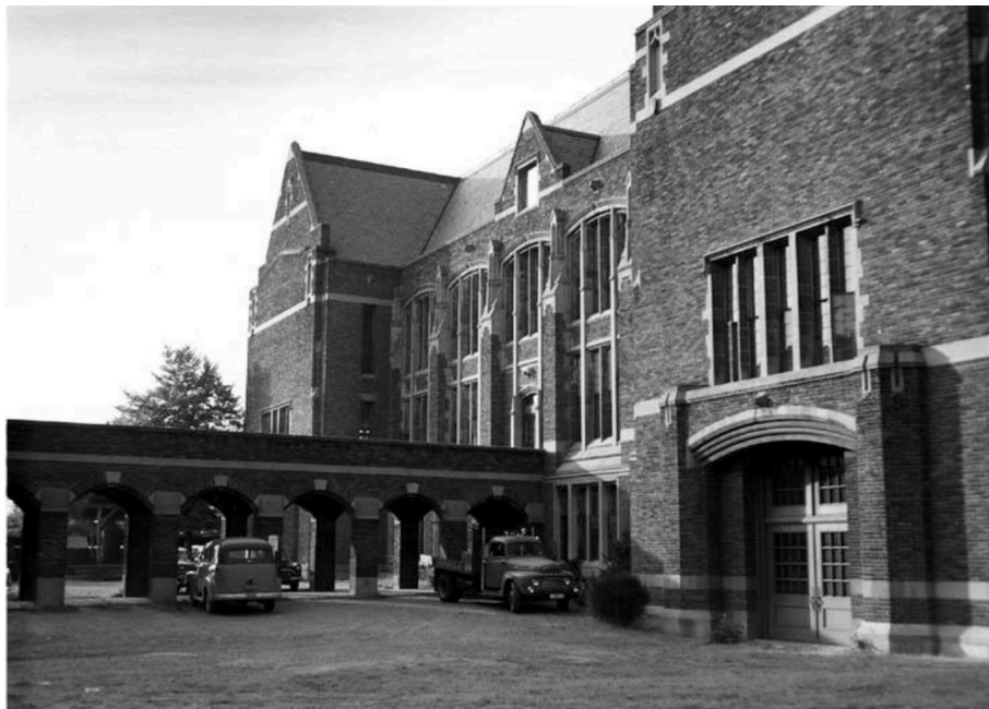
Figure 66. South face of Anderson Hall, showing the arcade that connected the main building to the Forest Products Lab, ca. 1940-1950. Source: University of Washington Libraries, Special Collections, Order # UWC3258.
