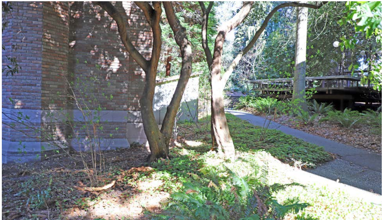
Figure 30. Southeast corner looking north along the east side of the building.
