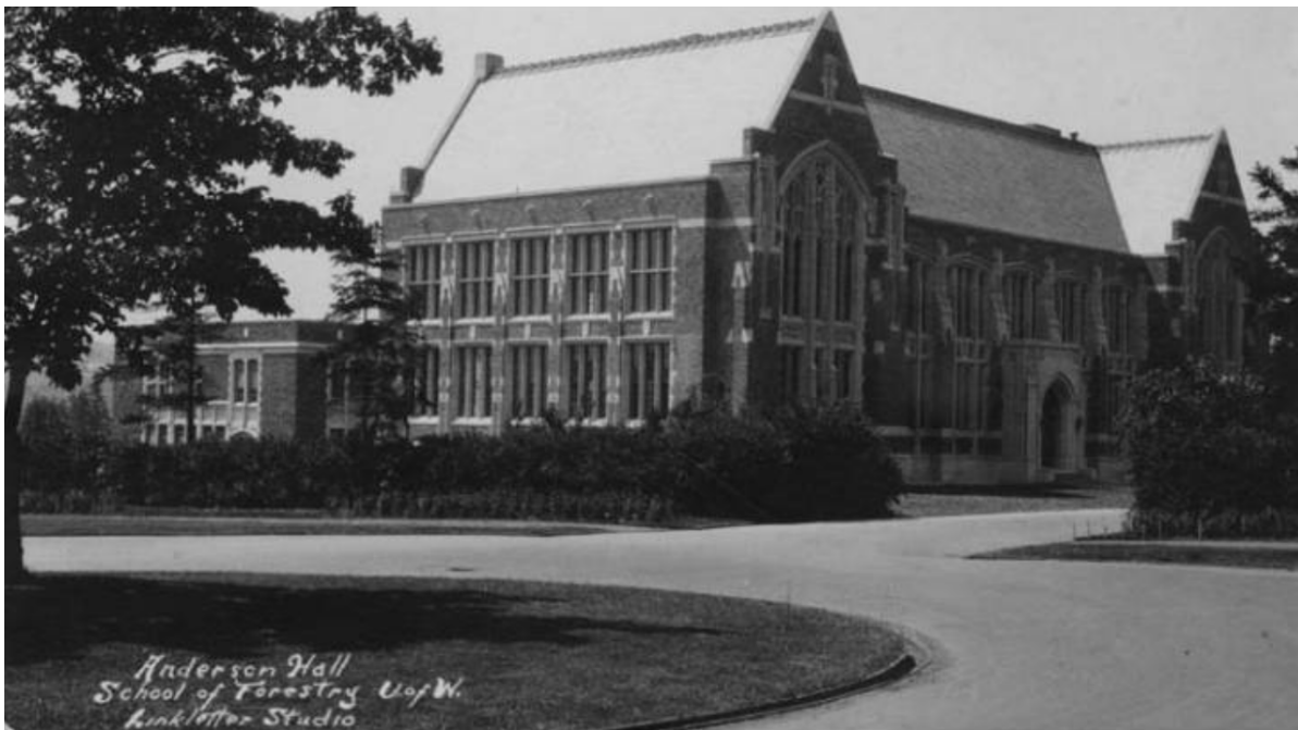
Figure 64. Anderson Hall, ca. 1925-1937, looking southwest along north and east facades.
