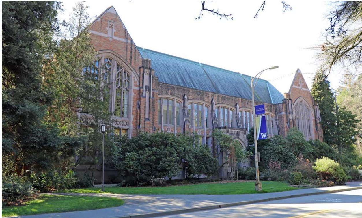
Figure 21. North facade, looking southwest.
