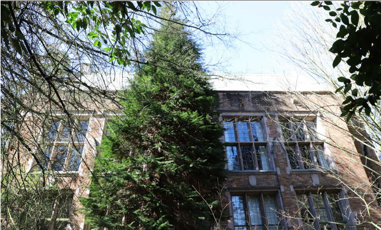
Figure 33. East facade, upper stories.
