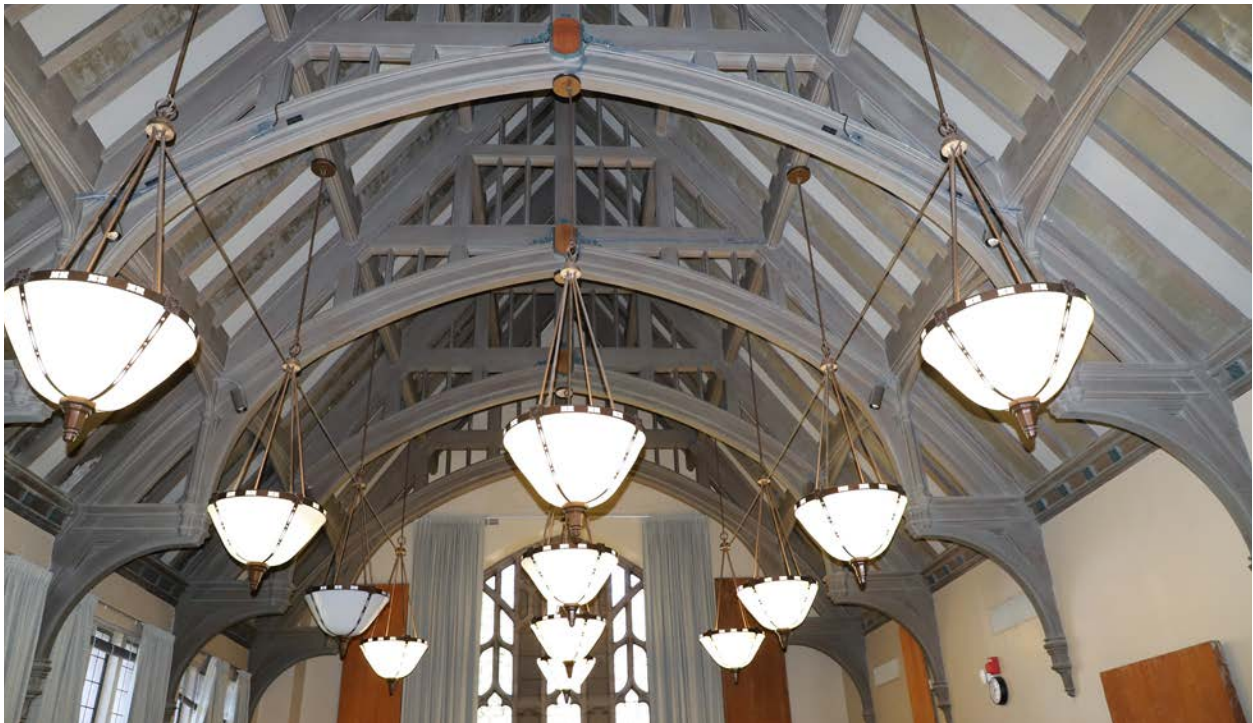
Figure 56. Lecture Hall, roof framing, looking north.
