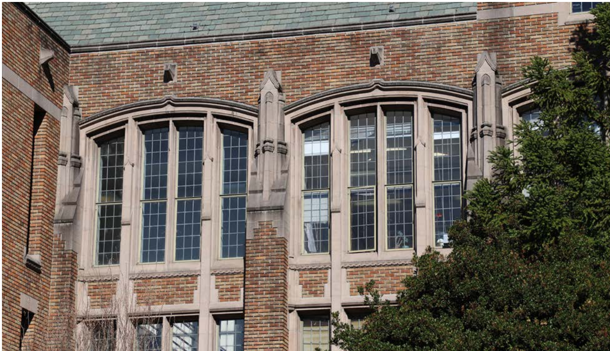
Figure 28. South facade, upper story detail.
