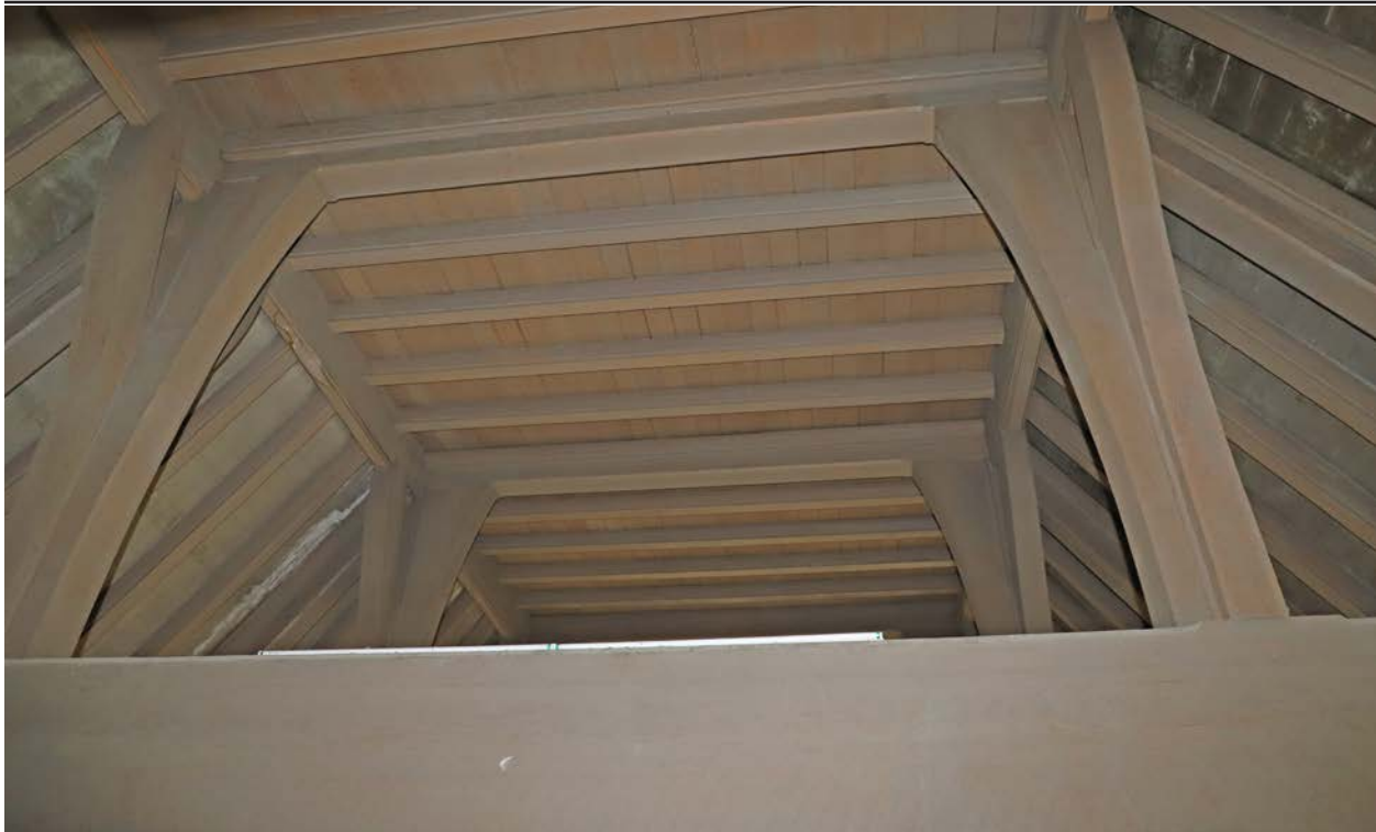
Figure 61. Reading room, roof framing.
