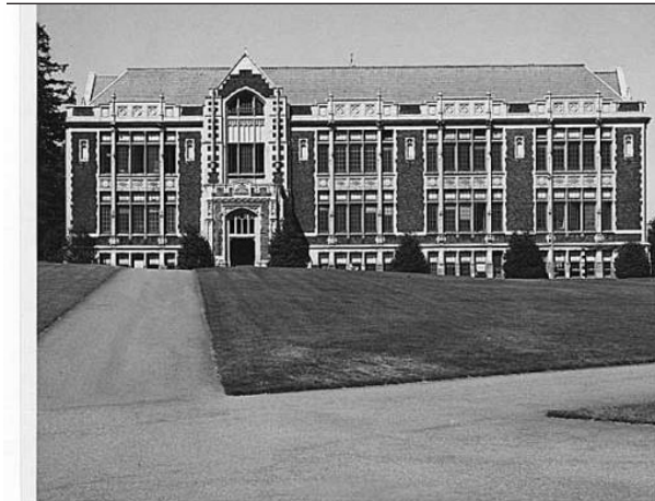
Figure 74. 1958 view of Savery Hall.
