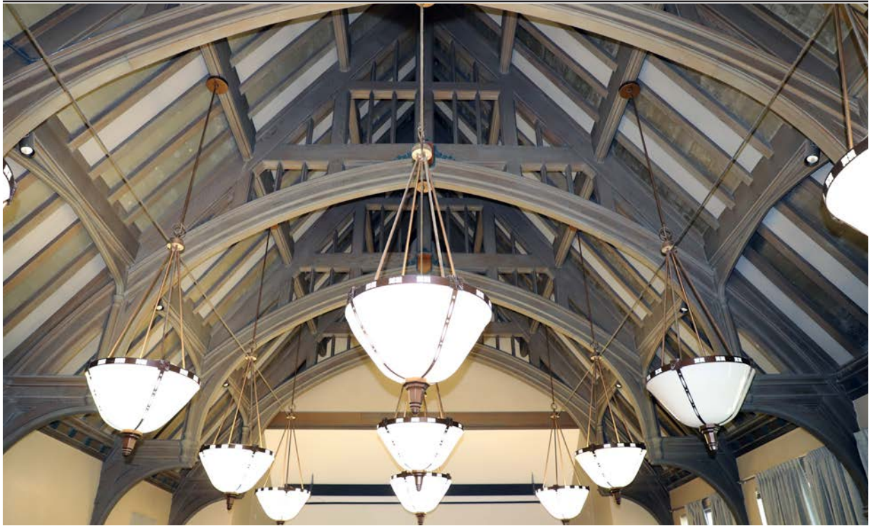
Figure 55. Lecture Hall, roof framing, looking south.
