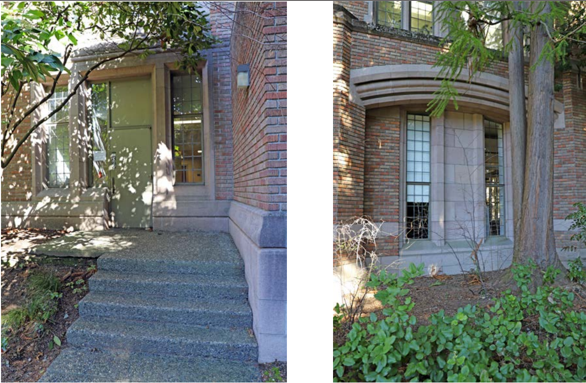
Figure 29. Southeast entrance (above left), and former south entrance converted to windows in 1968 (above right).
