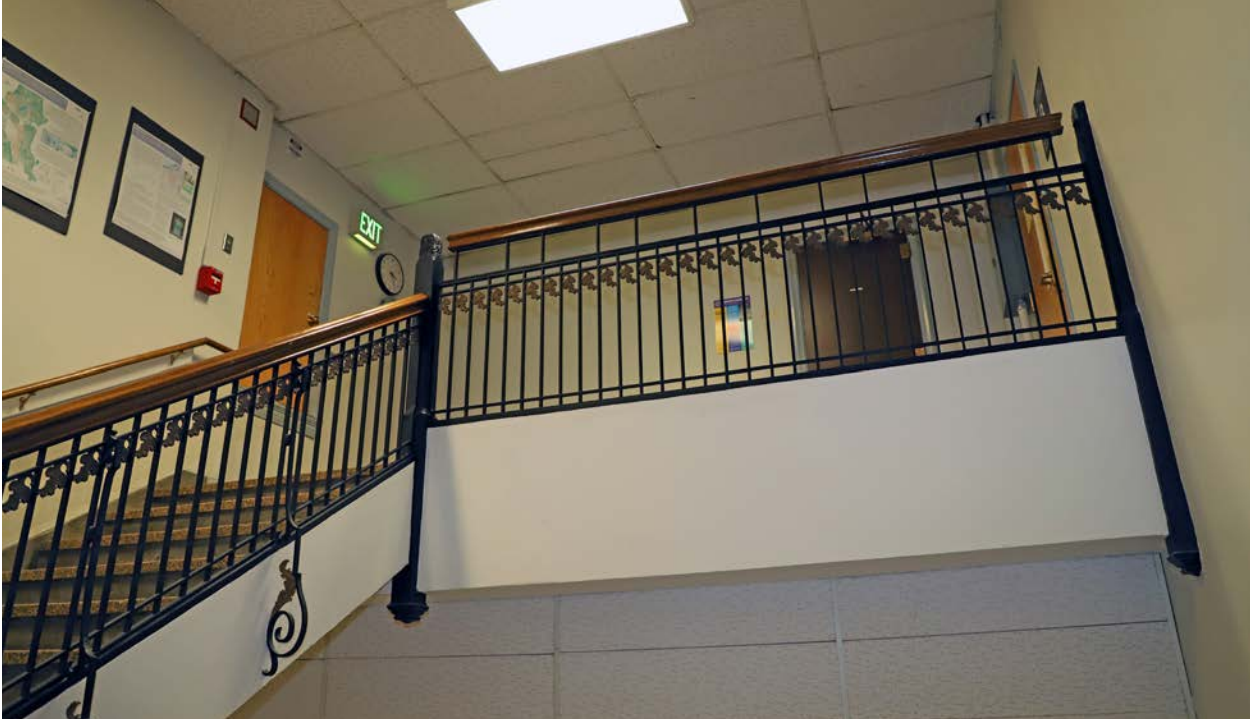
Figure 52. West stair, looking up to the third floor.
