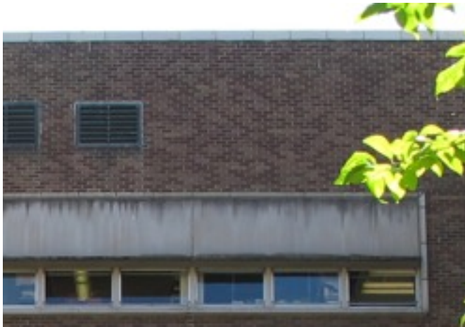
Existing façade-to-roof condition at roof B2.
