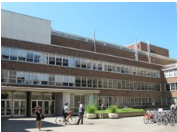
Entry courtyard created by A, C, D, and T wings.
