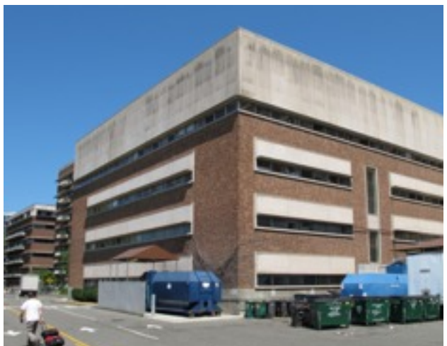
B wing seen from NE Columbia Rd.
