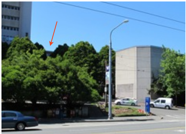
AA wing seen from NE Pacific St.
