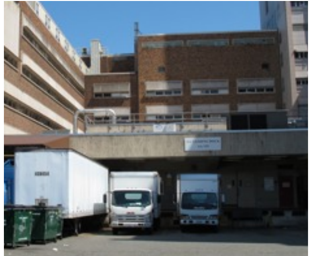
AA wing seen from NE Columbia Rd.
