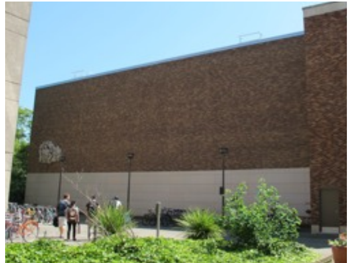
Minimal impact of metal railing set back from edge of roof.
