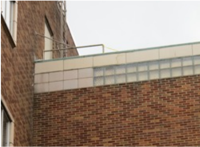
Existing façade-to-roof condition at roof C4.
