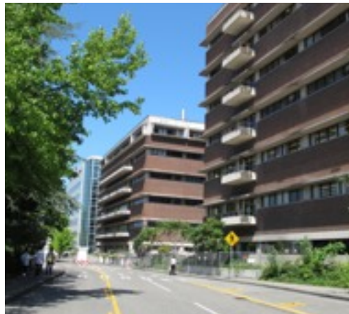
View along NE Columbia Rd.
