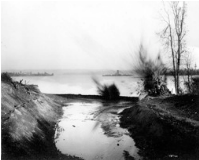
Opening the widened cut in 1910.
