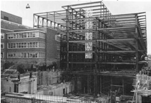
T wing under construction.
