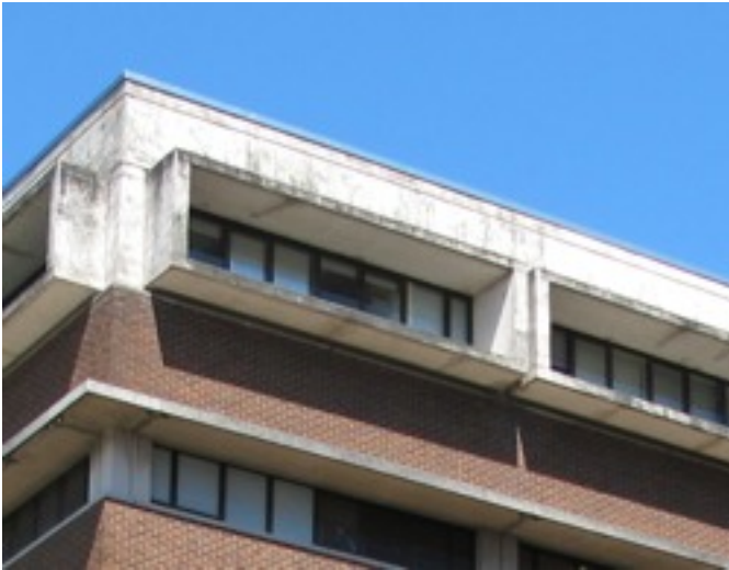
Existing façade-to-roof condition at roof F13.
