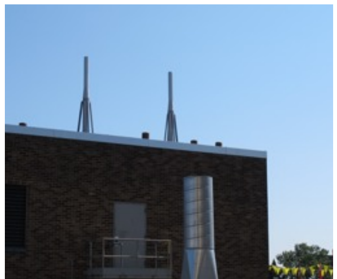
New and old vents on D5 visible from an adjacent roof.
