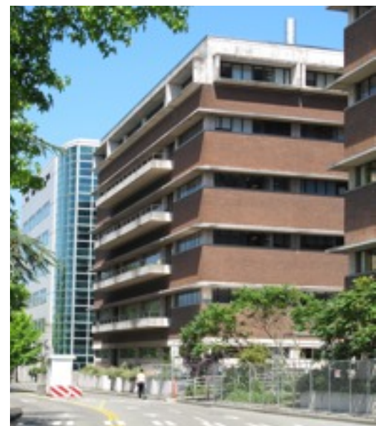
F wing seen from NE Columbia Rd.
