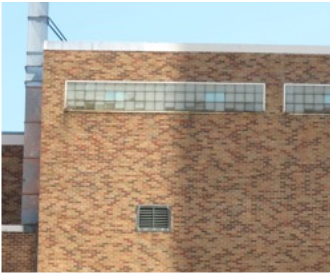
Existing façade-to-roof condition at roof AA.
